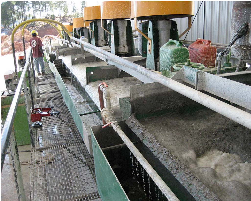
FLOTATION CIRCUITS AT CIENEGUITA
